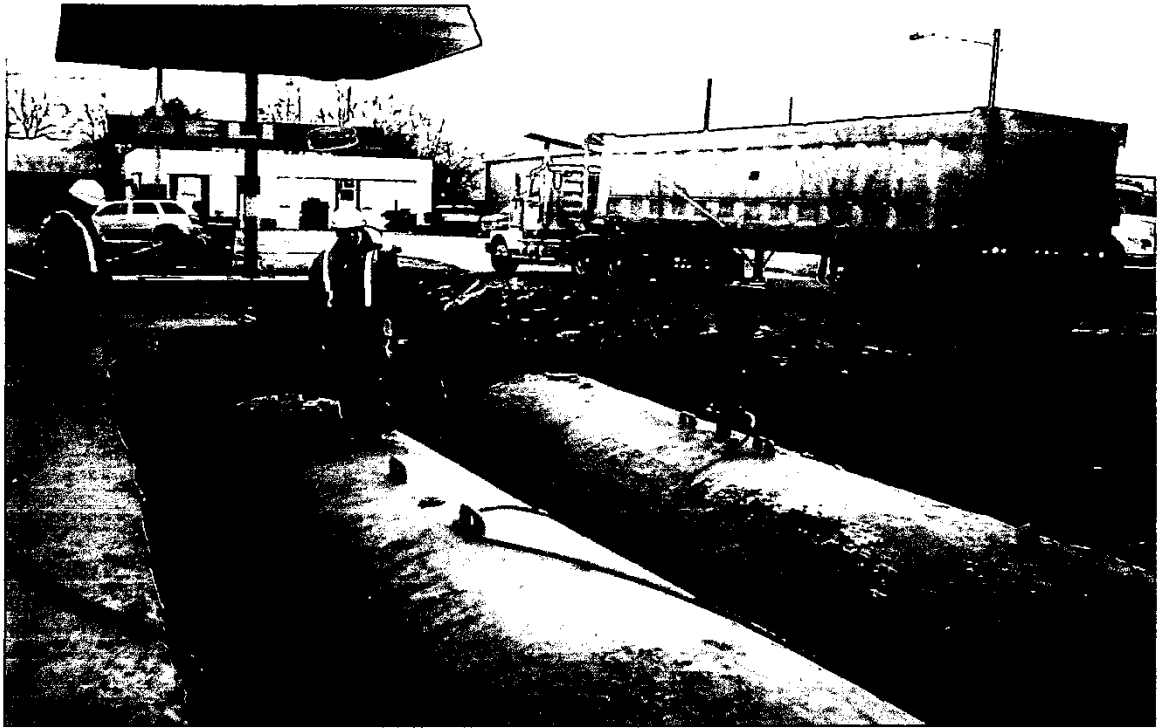
Tanks being purged prior to removal.
