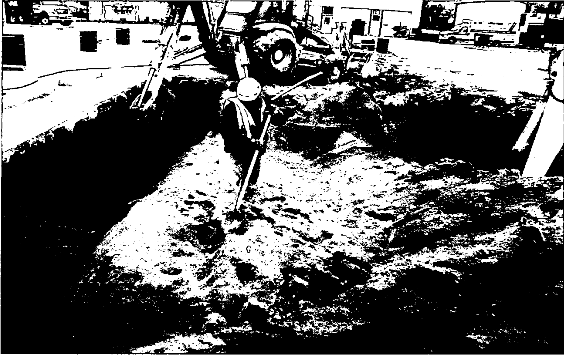
View of tank pit as backfill was cleared from UST's.
