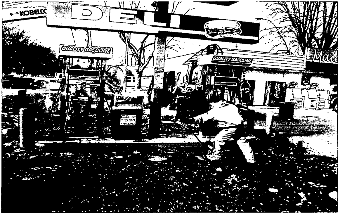
View of dispenser island prior to the removal of the pumps.
