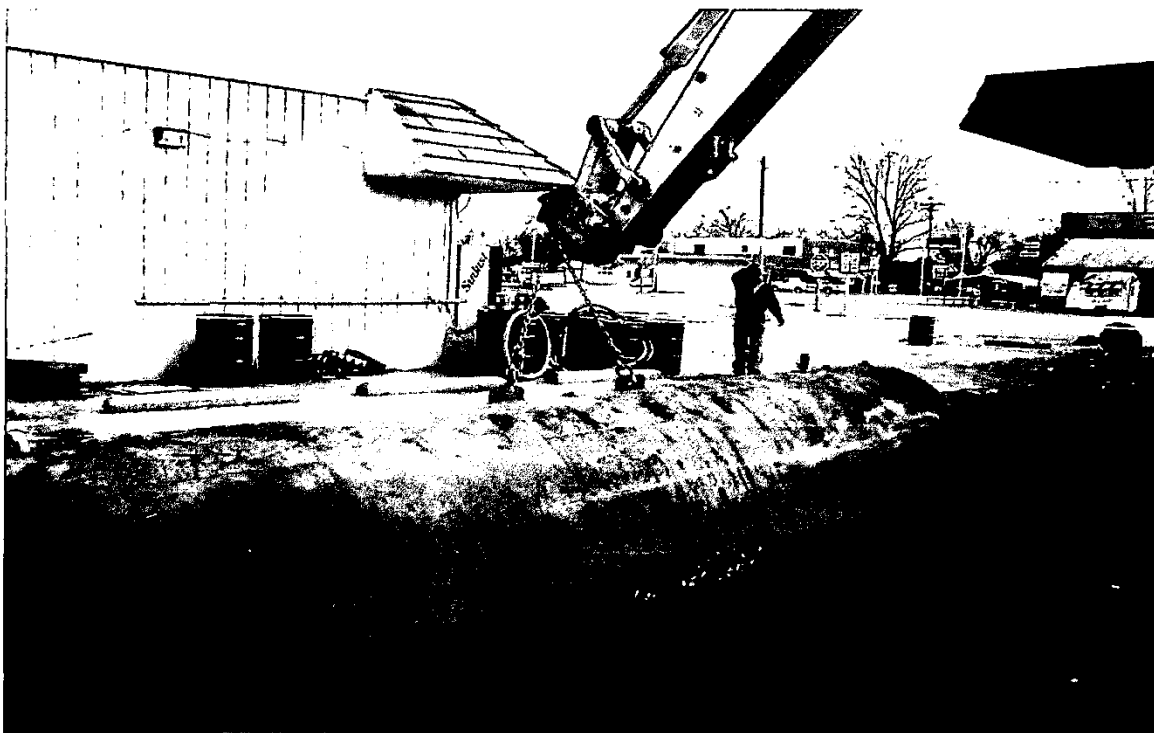
10,000 gallon UST lifted from tank pit.
