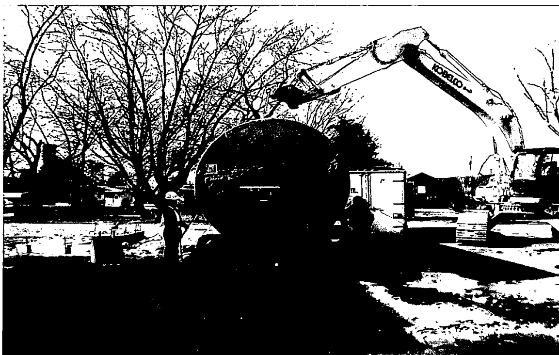
Cut and cleaned UST loaded for scrap.
