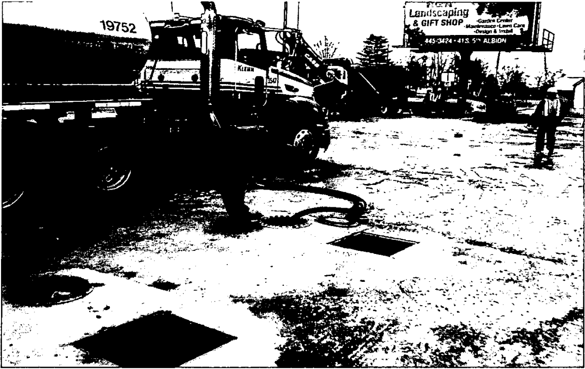
View of remaining fuel being removed from active UST.
