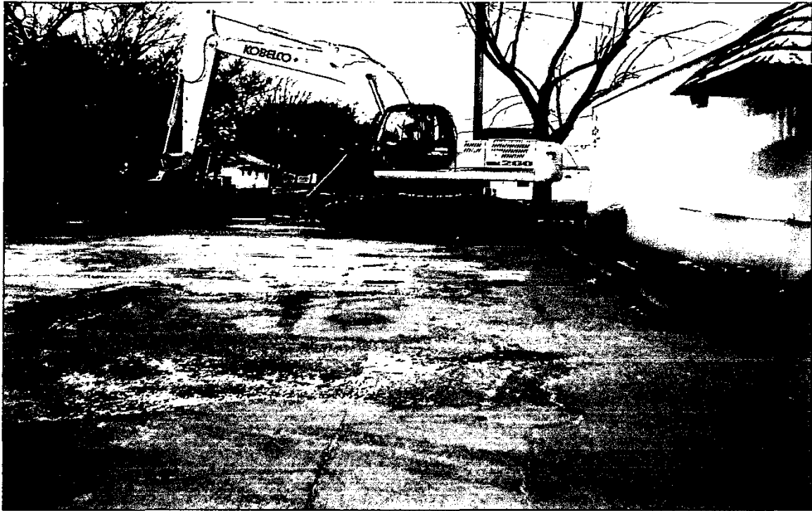
Tank pit prior to removal.
