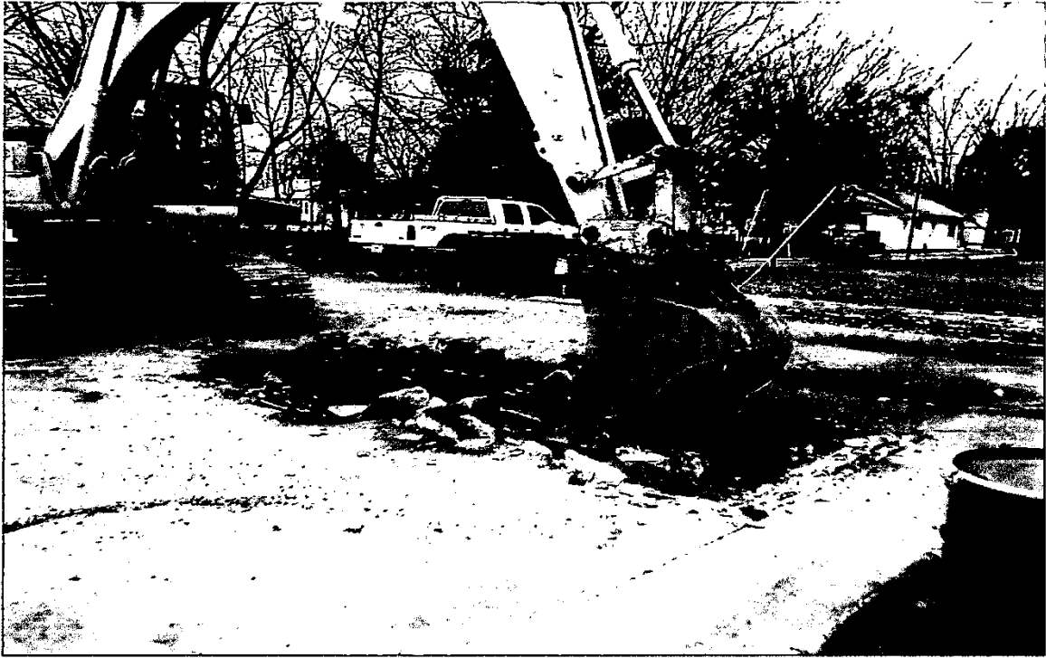
Commencement of concrete removal over UST pit.
